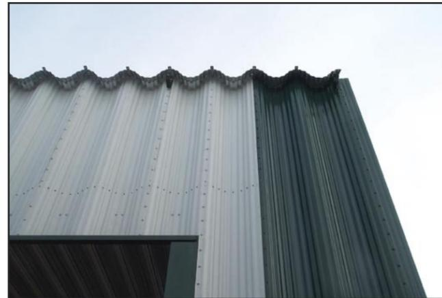
Manufactured from Galvanized or Galvalume™ steel in thickness ranging from 24 gauge through 13 gauge, this panel has a multitude of applications including roof panels and load bearing and non-load bearing wall panels. Available with or without precision punched side and end lap splice holes, our Frameless Panels can be installed in virtually any configuration.
